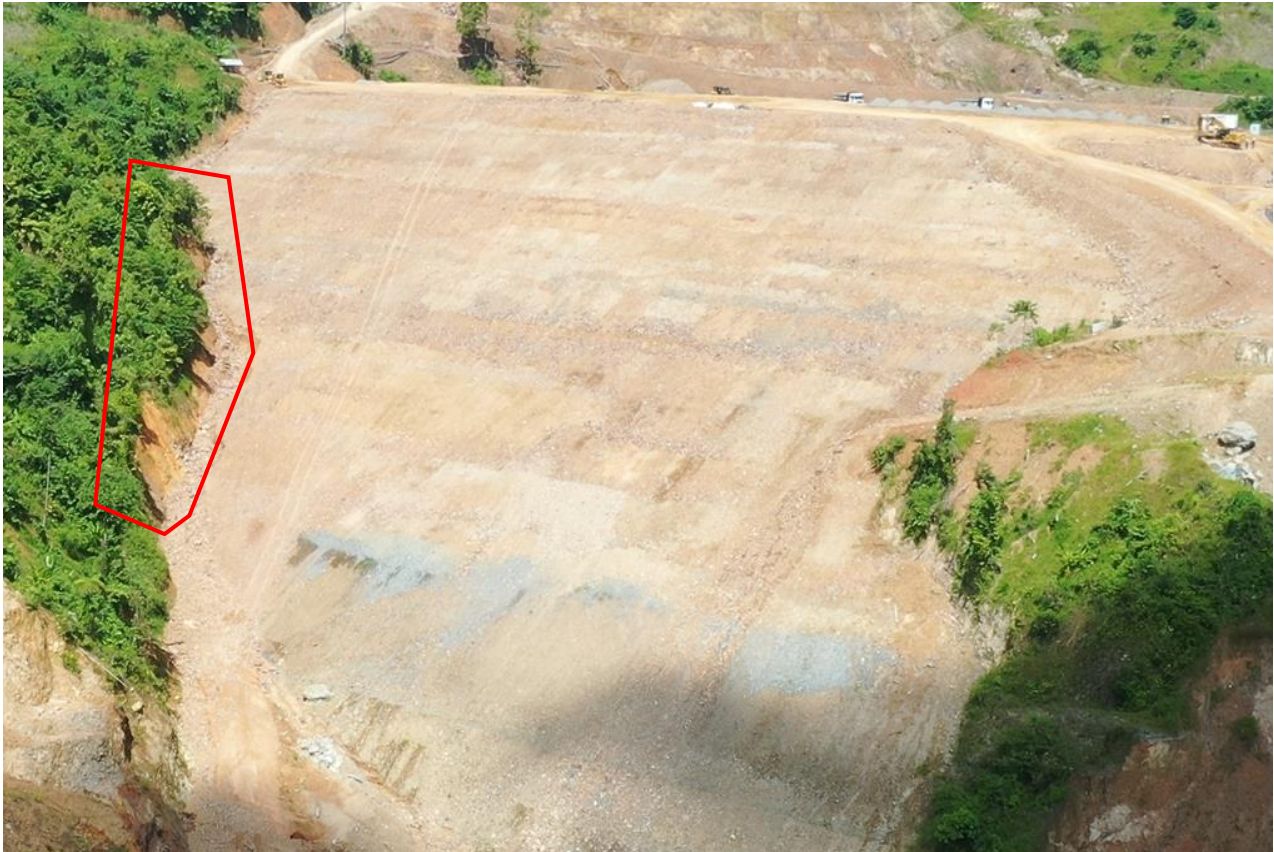
Figure 7 Significant erosion on right abutment
