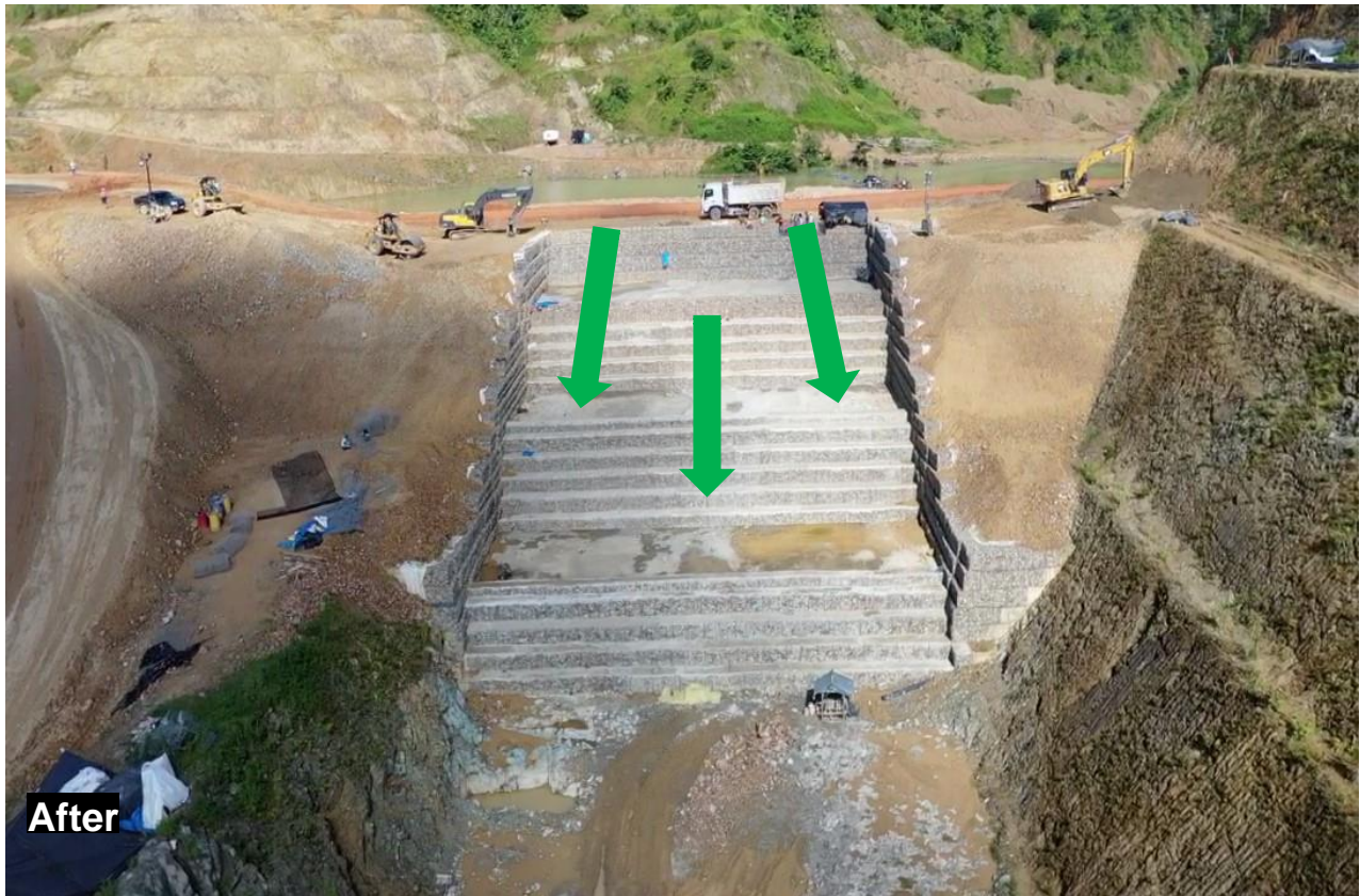
Figure 5 Properly constructed spillway
