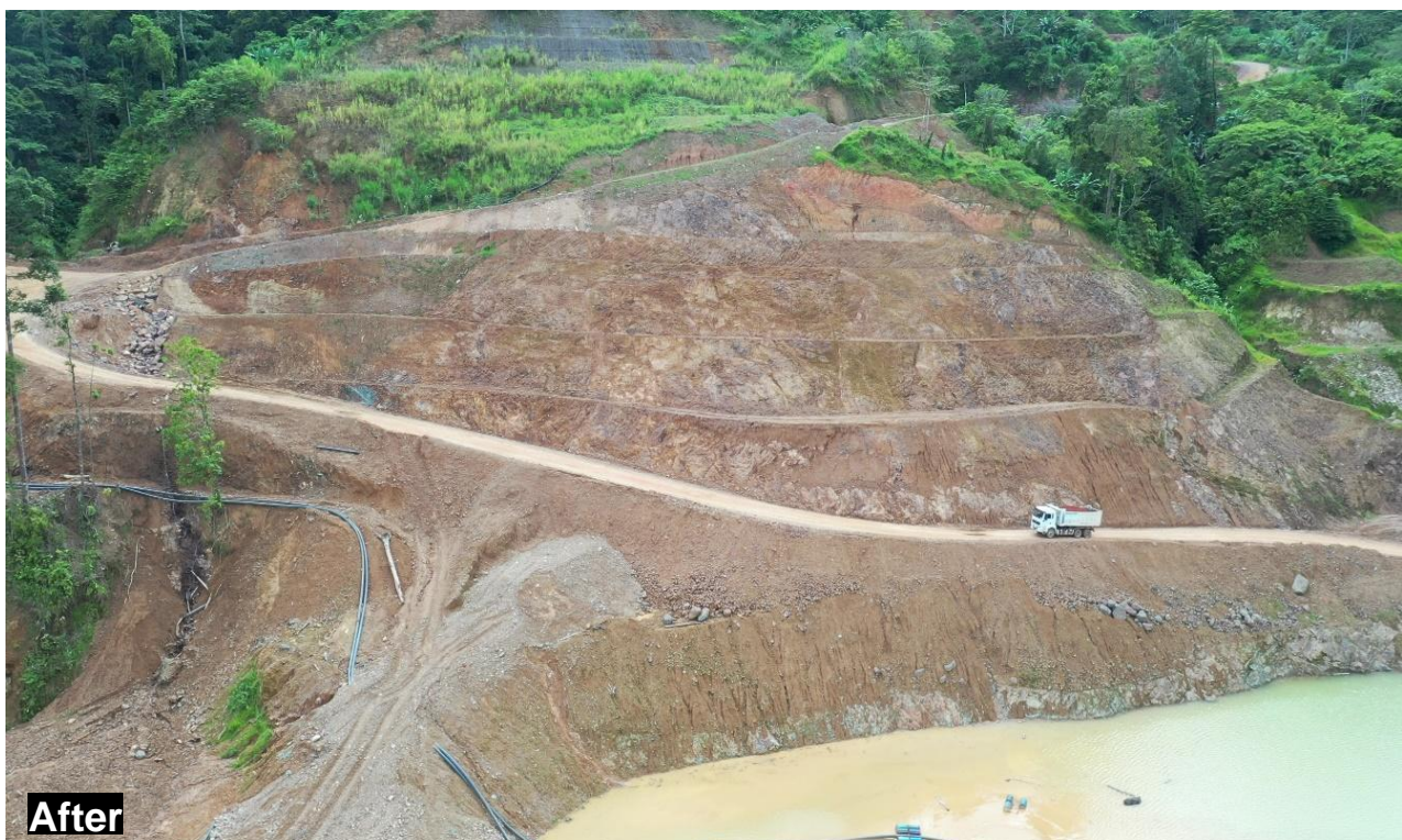
Figure 3 Batter after stabilisation works.
