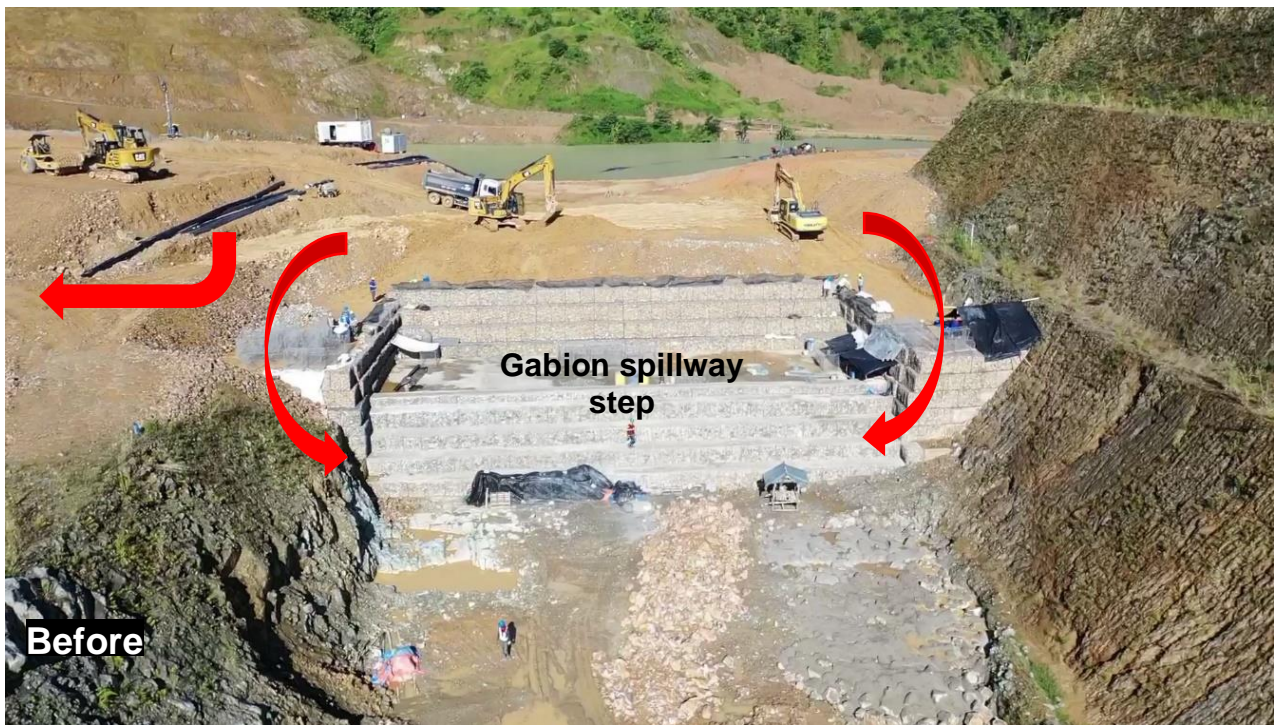
Figure 4 Gabion spillway walls lower than crest
