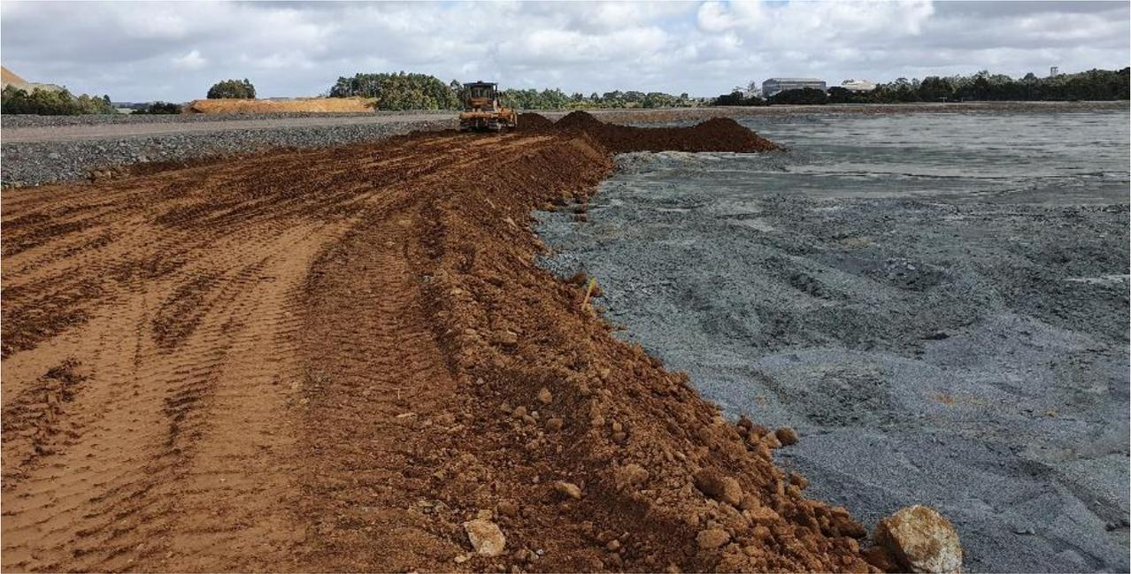
Figure 8 Clay cover placement.
