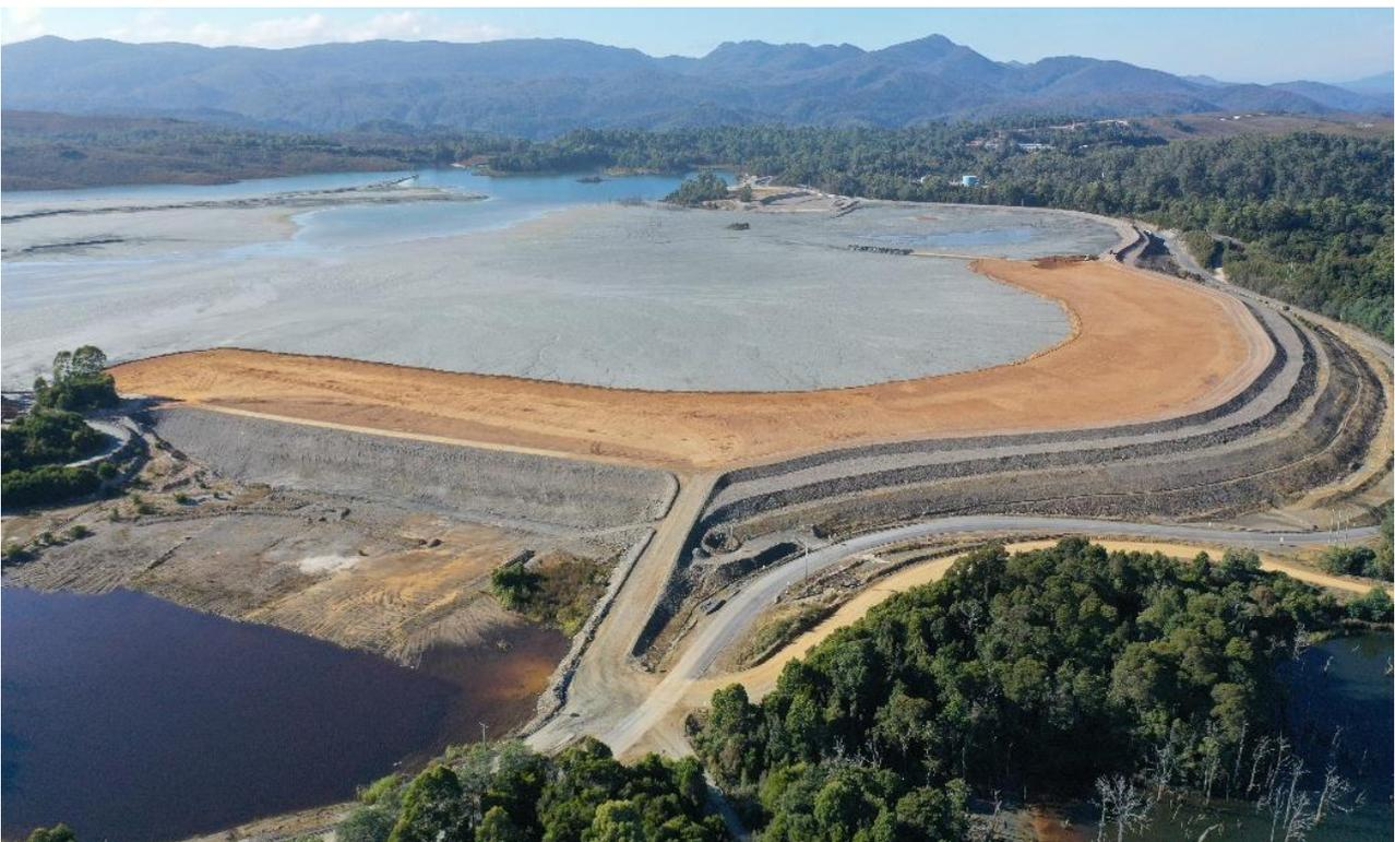
Figure 9 Clay cover placement.
