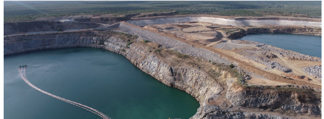
Kidston Pumped Hydro, Queensland
