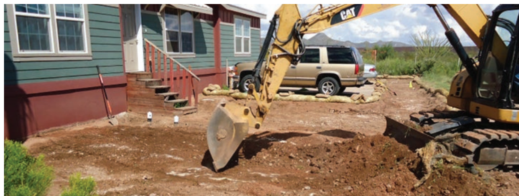
Townsite Smelter Program, property remediation, USA
