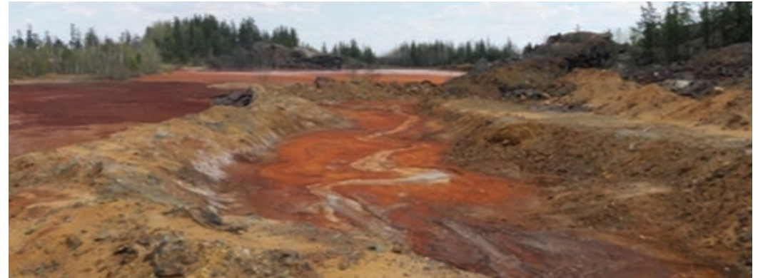
Kam Kotia Mine Site Reclamation, Canada
