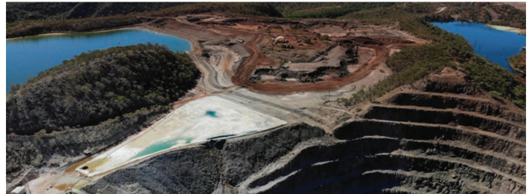
Clean Water Diversion
